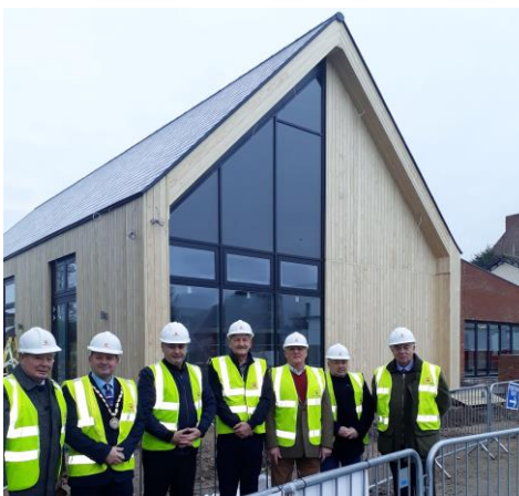
Tower Gardens Pavilion Construction
